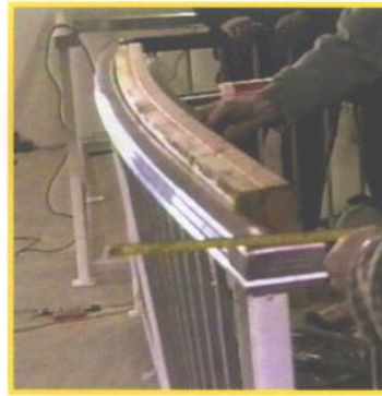
Picket Rail System Maximum Span - 10ft
